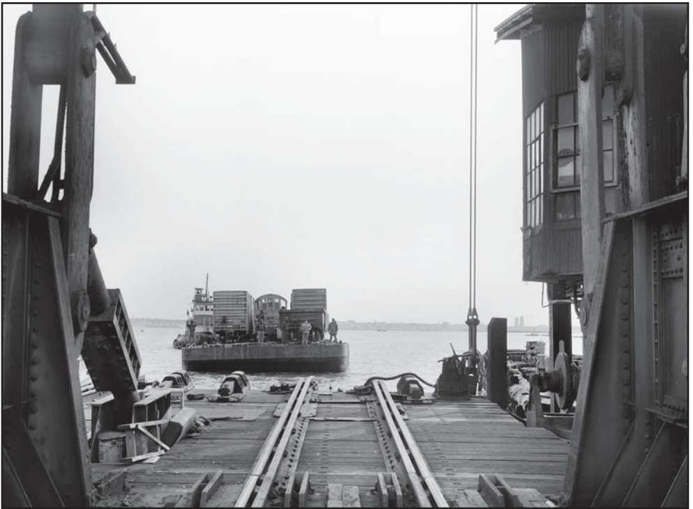
Eastward view of a loaded carfloat and tugboat approaching Transfer Bridge 11 of the Greenville Yard, winter 1996-97. This photograph and the photograph on the facing page were part of a 2011 Greenville Yard Transfer Bridge System HAER Recordation (Hayden 2011).
