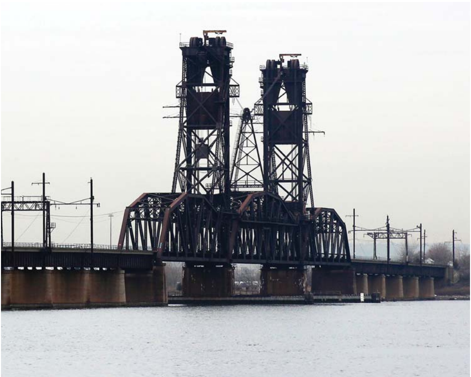
Westward view of the lift section of the PRRC and LVRRCNJ's Newark Bay Bridge, affording 135 feet of vertical clearance above the waters of Newark Bay. CHRS, Inc. photograph, January 31, 2020.
