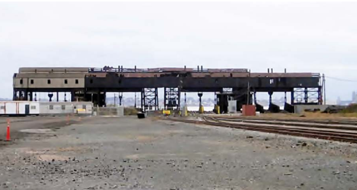
Eastward view of (from left to right) Transfer Bridges 9, 10, 11, and 12, circa 2011. From the 2011 Greenville Yard Transfer Bridge System HAER Recordation (Hayden 2011).
