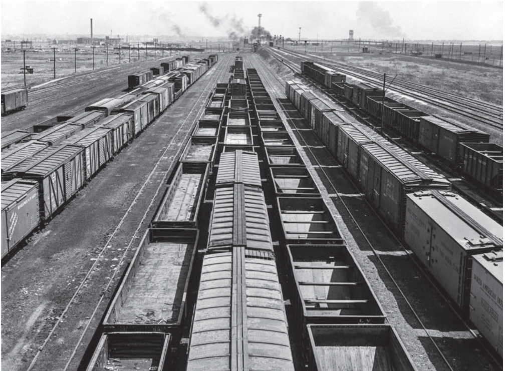
The Garden Yard inaugurated along the New York Bay Railroad's Greenville Branch in March 1939 appears in the upper right-hand corner of this eastward-looking photograph taken in April of that year. The LVRRCNJ's expansive Oak Island Yard fills most of the rest of the frame. When a five-track "New Garden Yard" was installed to the west (behind the photographer and out of frame) in 1943, the compact Garden Yard was renamed "Old Garden Yard." (Library of Congress)
