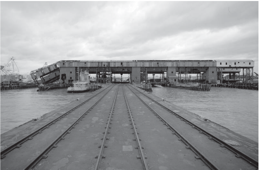
Westward view of the Greenville Yard Transfer Bridge Assembly, 1996 (Louis Berger & Associates, Inc. 1996).
