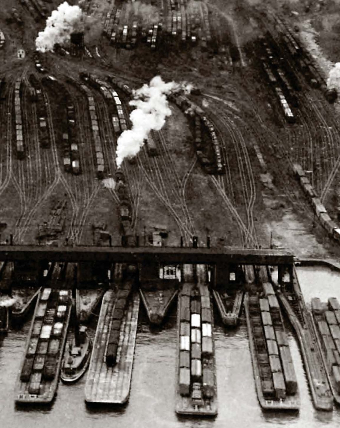
Westward aerial view of transfer bridges at the eastern end of the Greenville Yard on the Pennsylvania Railroad Company's New York Bay Railroad, from the 1949 pamphlet Pennsylvania Railroad Harbor Facilities: Port of New York.
